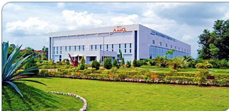
Works at Nagpur
